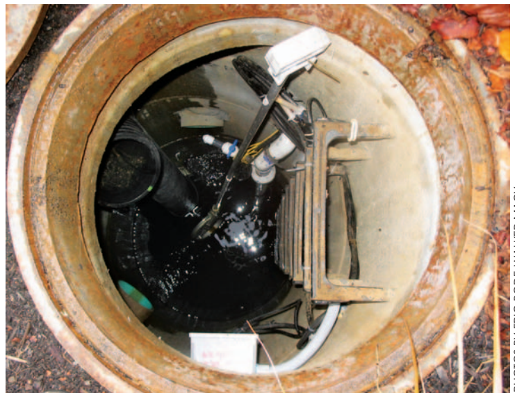
ABOVE: The water collection system utilizes a traditional storm pipe for collection and distribution to the overall campus system. The T-handle at top closes an overflow gate that can be left open to drain excess rainwater when the collecting pond is full.
