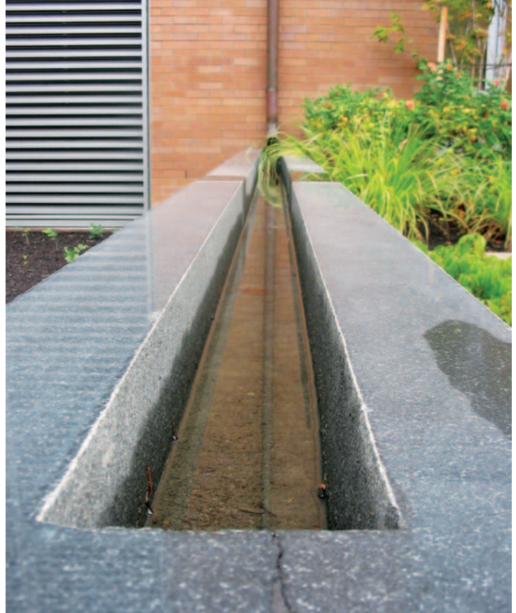
ABOVE: Some of the aqueducts spill from the ends, others from the center (the outflow is at center right here). The water channel runs the length of the water-quality garden to create an eye-pleasing line.
