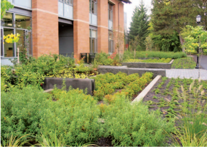
ABOVE: Storm water planters line both sides of the building's entrance. The rectangular structure in the planting bed is an aqueduct that channels roof runoff to the bed. The runoff feeds dwarf red twig dogwood, which has a wide tolerance for dry and wet conditions.
