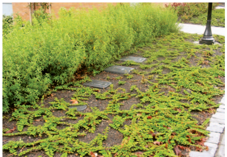
BELOW: The Landscape Architect paid careful attention to minimizing the visibility of irrigation equipment. The black valve boxes in the newly-planted beds are nearly invisible and will be completely hidden when the vegetation fills in.
