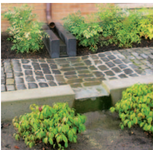
ABOVE: Storm water planters line both sides of the building's entrance. The rectangular structure in the planting bed is an aqueduct that channels roof runoff to the bed. The runoff feeds dwarf red twig dogwood, which has a wide tolerance for dry and wet conditions.
