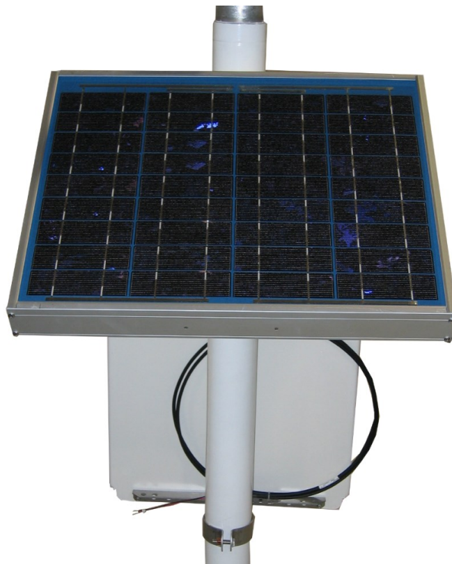
FIGURE C-9. Fully mounted solar panel
