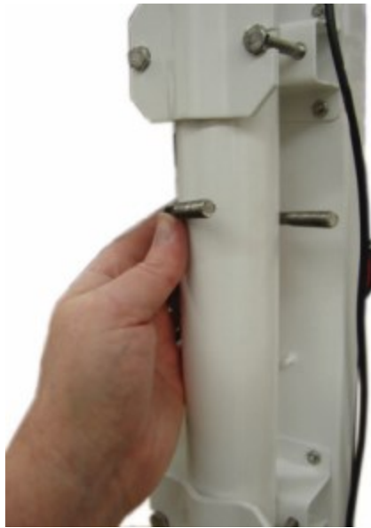
FIGURE 6-30. Slide antenna bracket U-bolt around back of the pole
