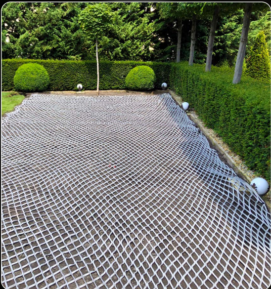
NET INSTALLATION ON A SECTION OF LAWN
