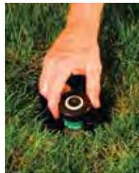
**2** Unscrew the old head. TIP: Check the threaded riser or other connector under the head. If it is also damaged, remove more soil to expose the entire fitting. Replace with with proper fitting thread and length.
