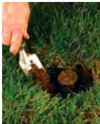
**1** Turn off water to the zone and carefully remove dirt around the sprinkler. Take care in not damaging any underground pipe or fittings.
