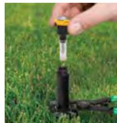
**3** Purchase a new nozzle with proper pattern and throw distance. See selection guide, page 7. Insert new filter screen screw on the new nozzle. (Hand tighten only.)
