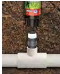
**3** Clean the threads and apply Teflon® tape to the male connector. Then screw on the new head.
