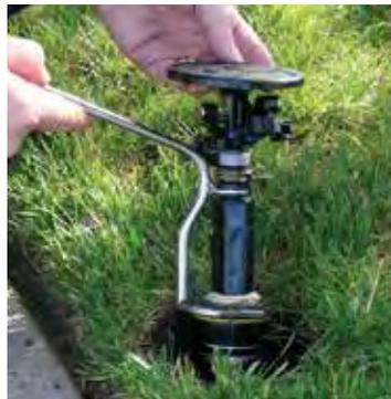
Replace the internal mechanism of in-ground impact sprinklers without digging.
