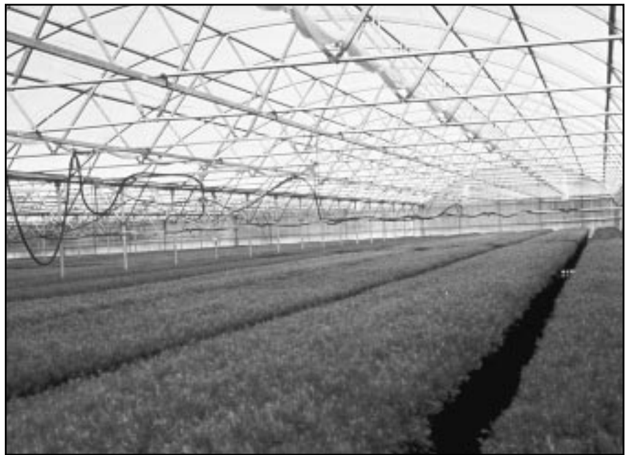
Greenhouse application with many short on-cycles during an irrigation “window”.
